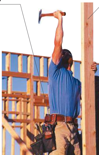
el albañil construction worker
