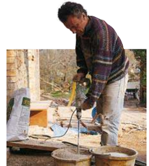
el albañil construction worker
